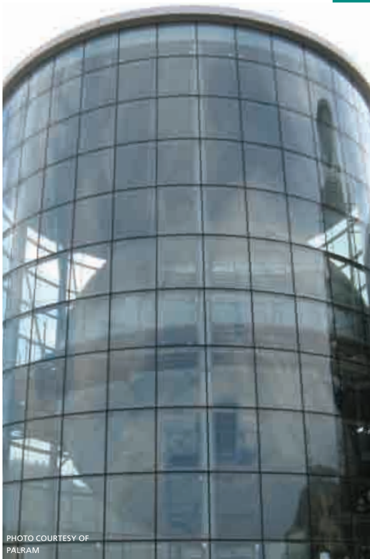
CURTAIN WALLING AROUND ROTATING RESTAURANT
